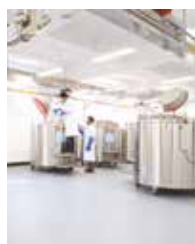
Chemical Storage Areas
